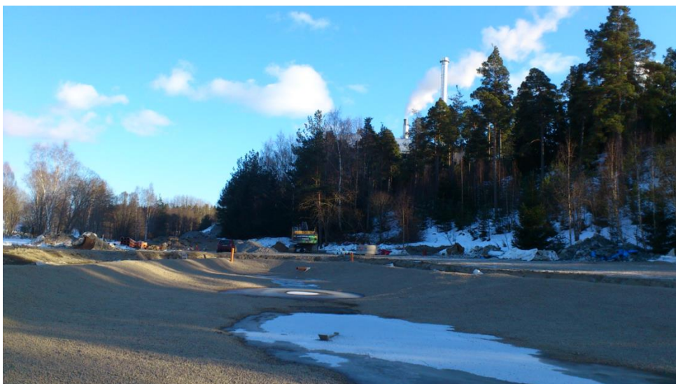
Figure 11 Fortum Dam Construction 2013-03-10, chimneys visible in the background (M Norling)
